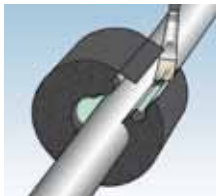
2 - Spread K-FLEX adhesive onto the half-collars.
